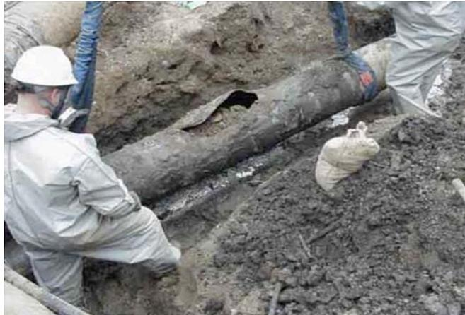
Figure 1.1 Actual rupture in the pipeline
