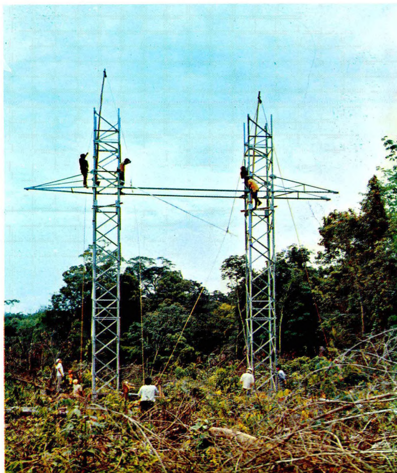
132 kV Transmission Line between Kuala Lumpur and Bentong Under Construction
